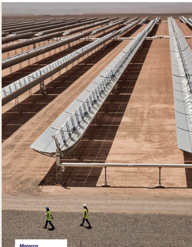
Morocco Noor Solar Complex
