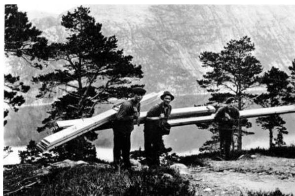
Hydropower construction work Lysefjorden in 1916
