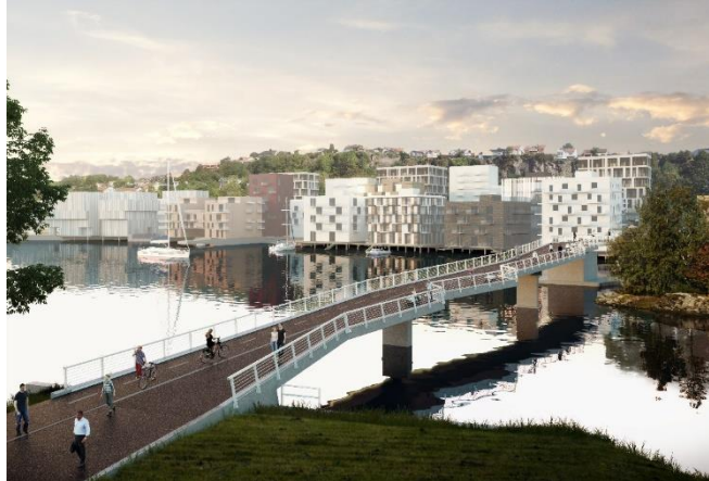
Pedestrian and cycling bridge to be built between Klosterøya and Jernbanebrygga in Skien as part of Bypakke Grenland. The bridge can be opened to allow for passing of larger boats.
