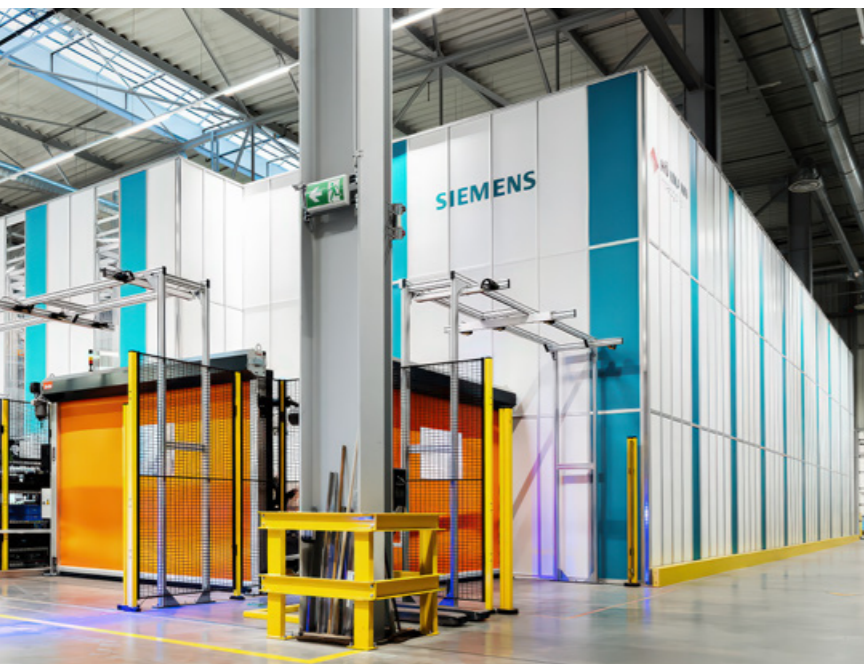
External view of the picking robot cell and AutoStore® system
