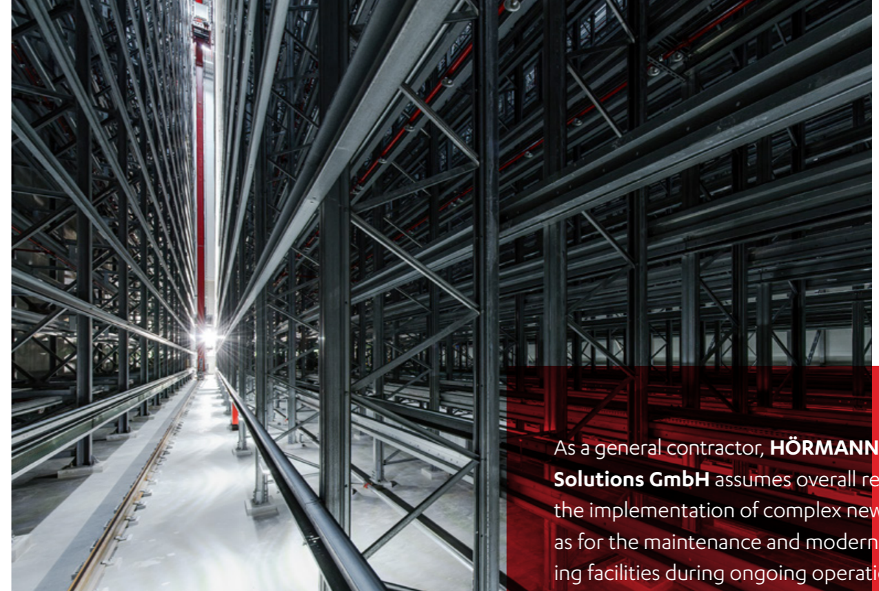
^ Inside the high-bay warehouse
