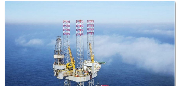
The jack-up drilling rig Borr Gerd
