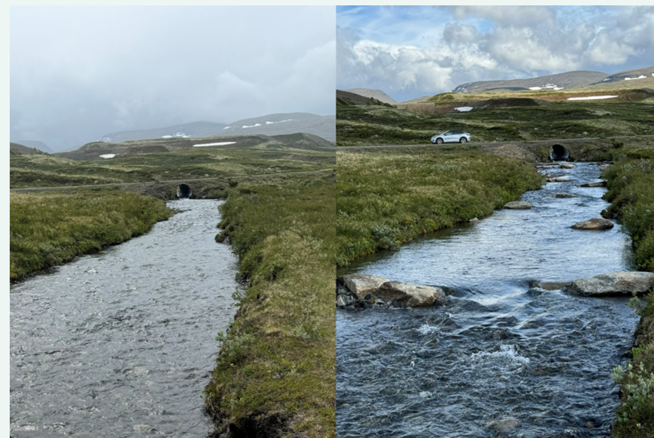
Before (left) and after (right) rock laying in the upper parts of the project area.
