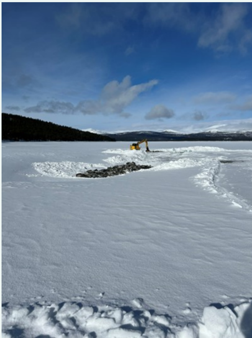
The image shows rock laying in the regulating zone in Savalen
