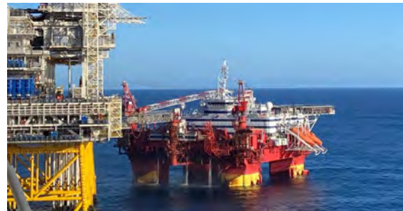
Floatel Endurance at the Johan Sverdrup, Phase II project.
