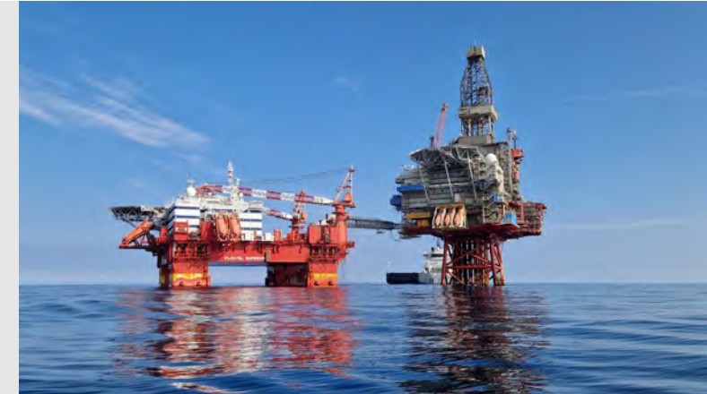
Floatel Superior commenced operation for Vår Energi at Ringhorne on the Norwegian continental shelf in July
