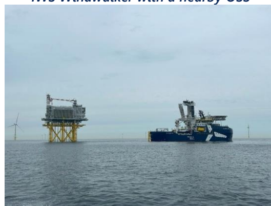
IWS Windwalker with a nearby OSS
