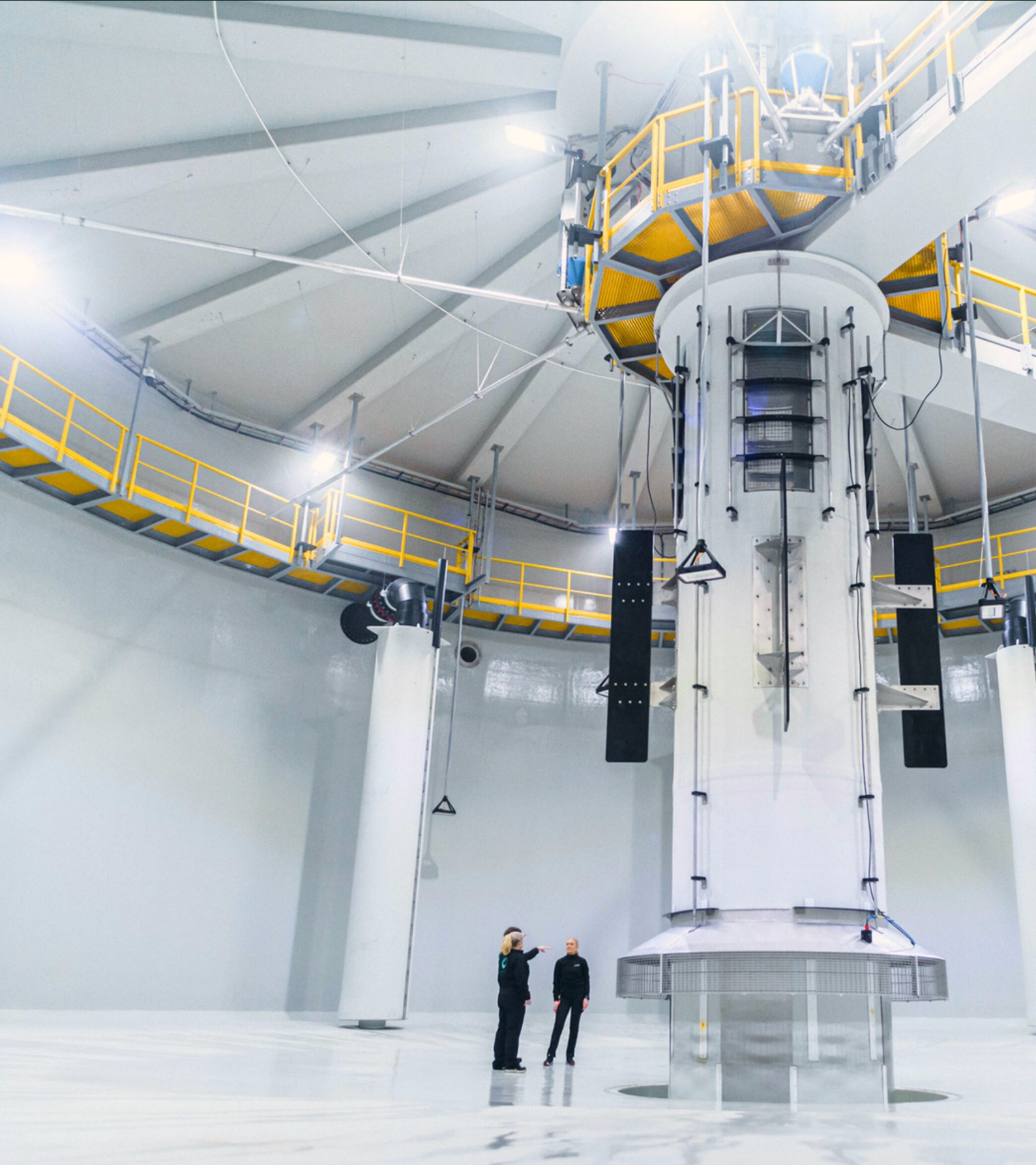
Empty fish tank at Salmon Evolutions grow-out facilities at Indre Harøy, where Artec Aqua AS was the turnkey supplier.
