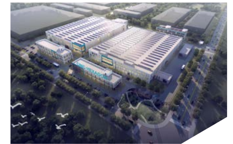
Shijiazhuang China Under construction
