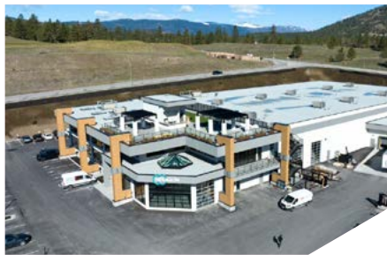
Kelowna Canada Construction completed
