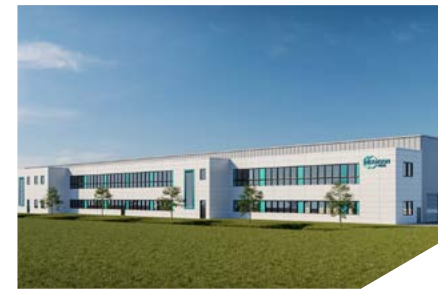
Weeze Germany Under construction
