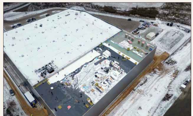
Oribalt | Expansion area under construction (end of 2022)
