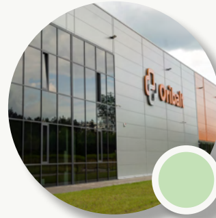
Oribalt terminal Status: Ongoing
