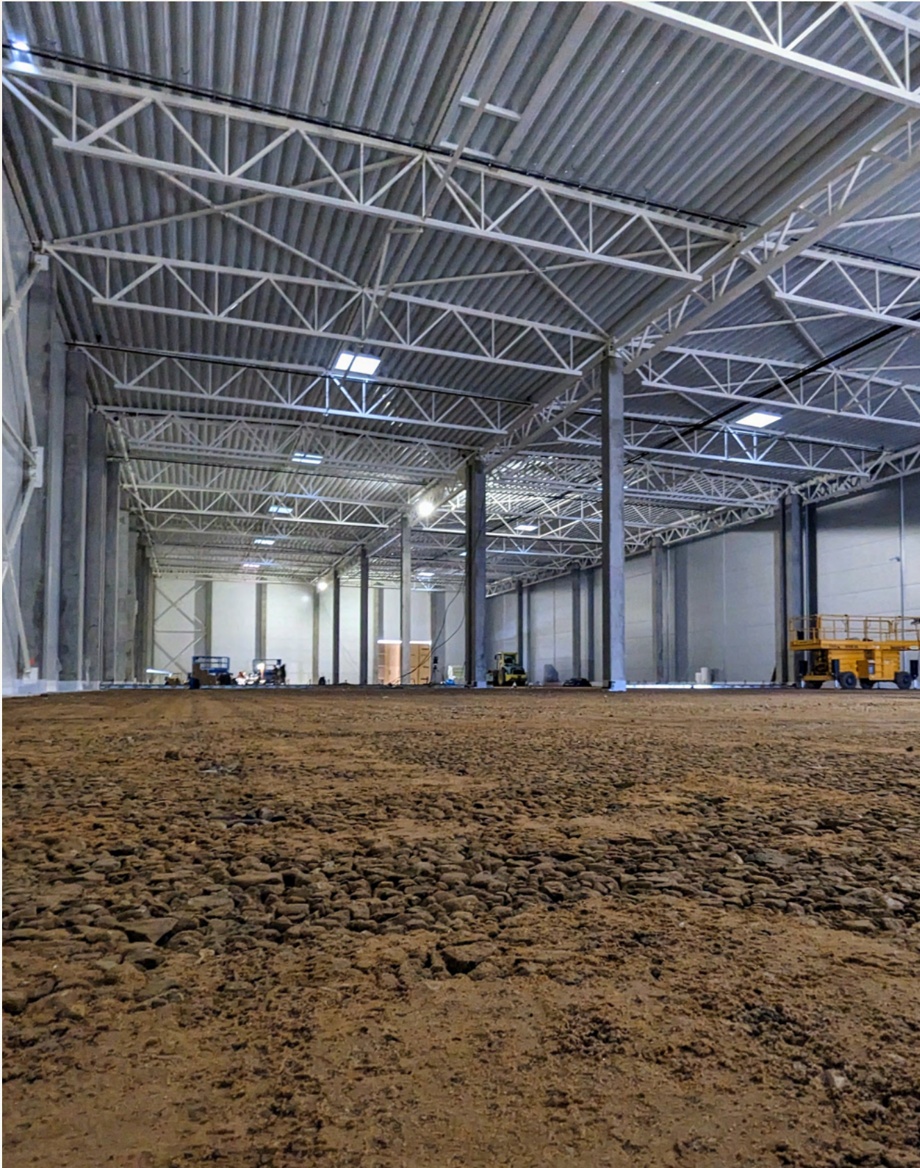
Oribalt | Expansion area under construction (November 2022)
