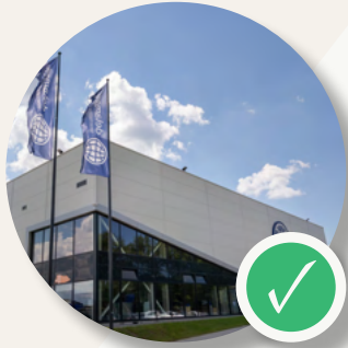
Delamode terminal BREEAM In-Use: "Very good"
