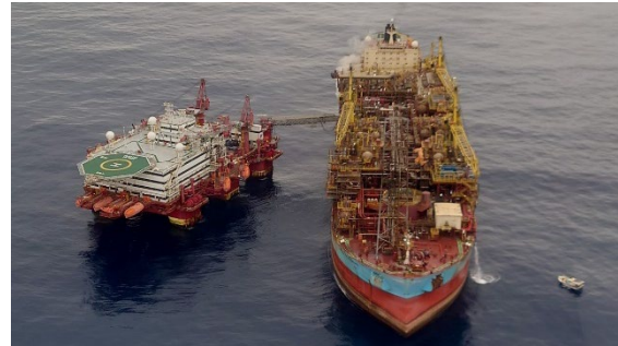
Floatel Victory is in operation alongside Peregrino FPSO.
