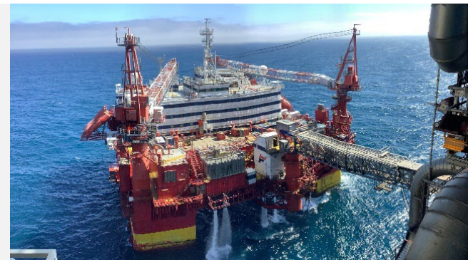
Floatel Superior on charter at Equinor's Breidablikk Project
