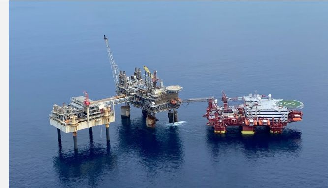
Floatel Triumph in operations for Shell at the Malampaya field in the Philippines
