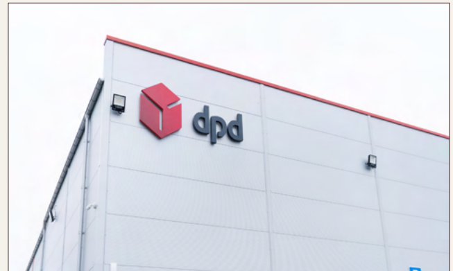
DPD | Completed in October 2022
