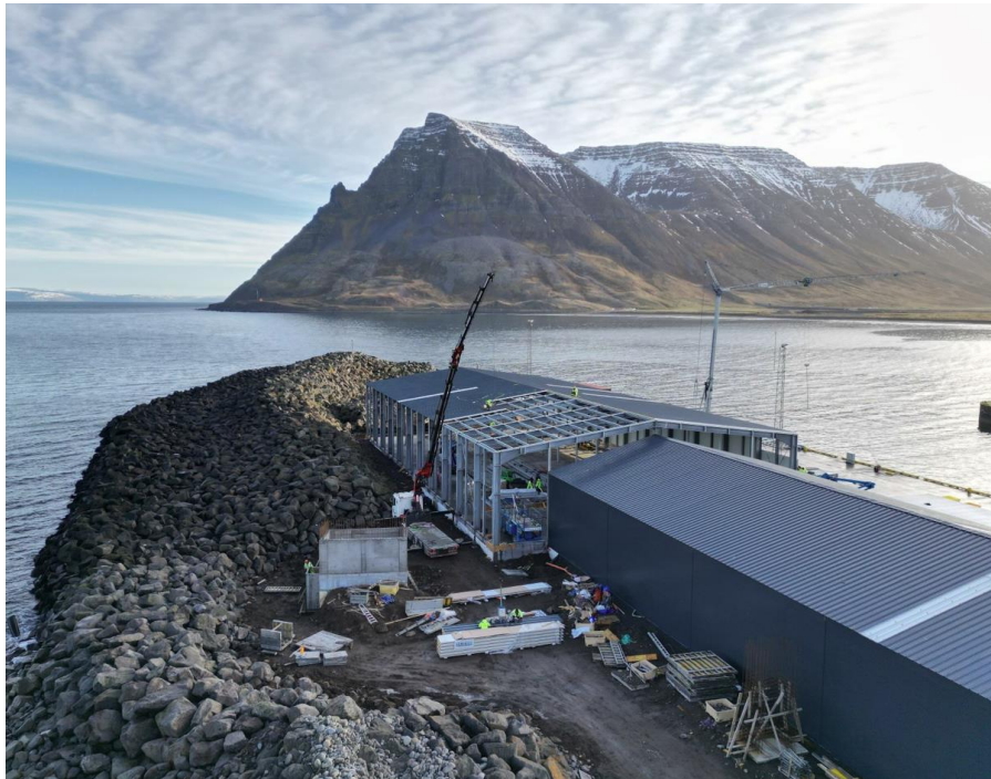
Harvesting facility building in Bolungarvík
