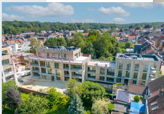
CFE > The Arboreto project in Tervuren, Belgium
