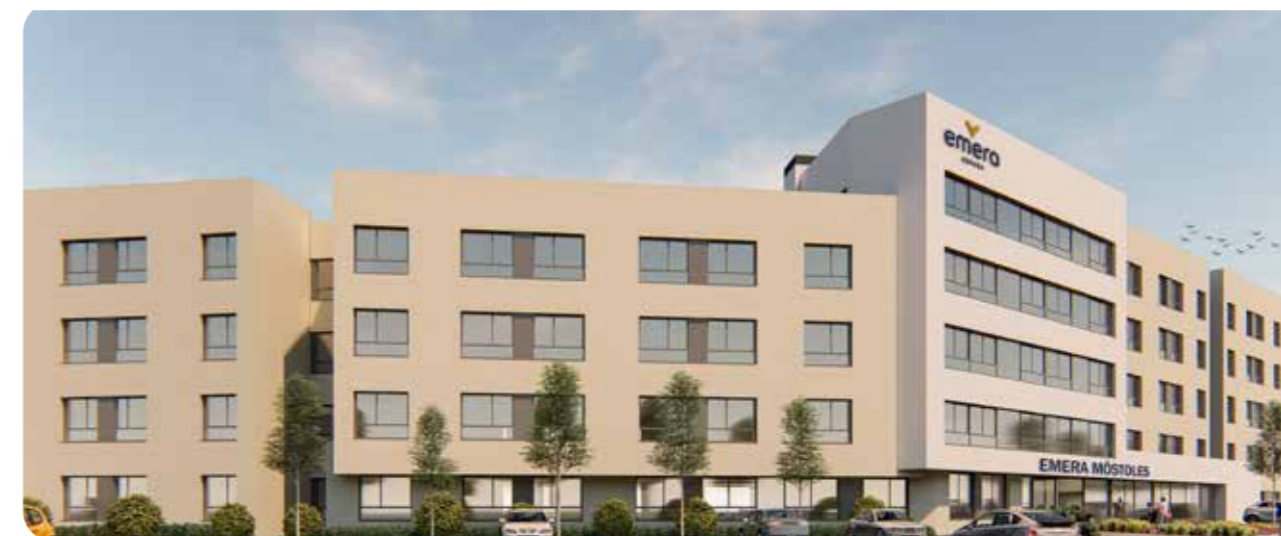
Mostoles (ES) | Emera Mostoles
