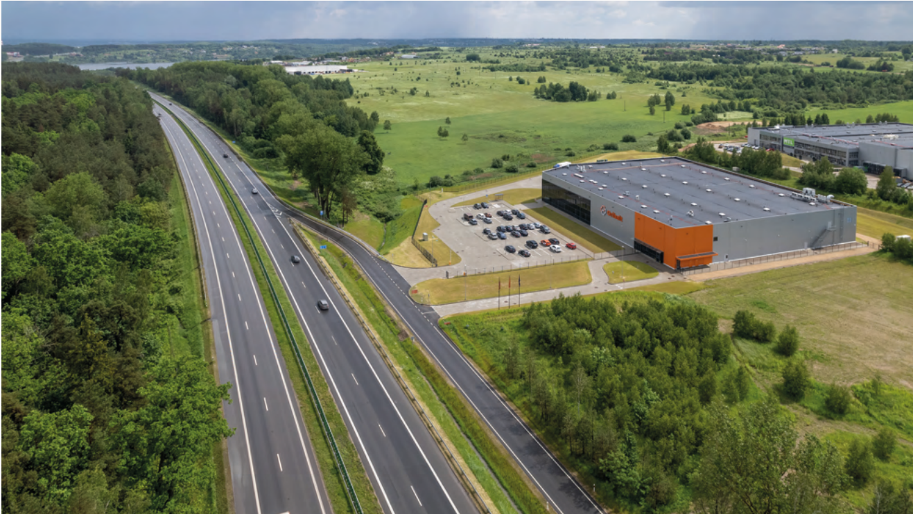
Oribalt terminal | Highway A1, near Vilnius
