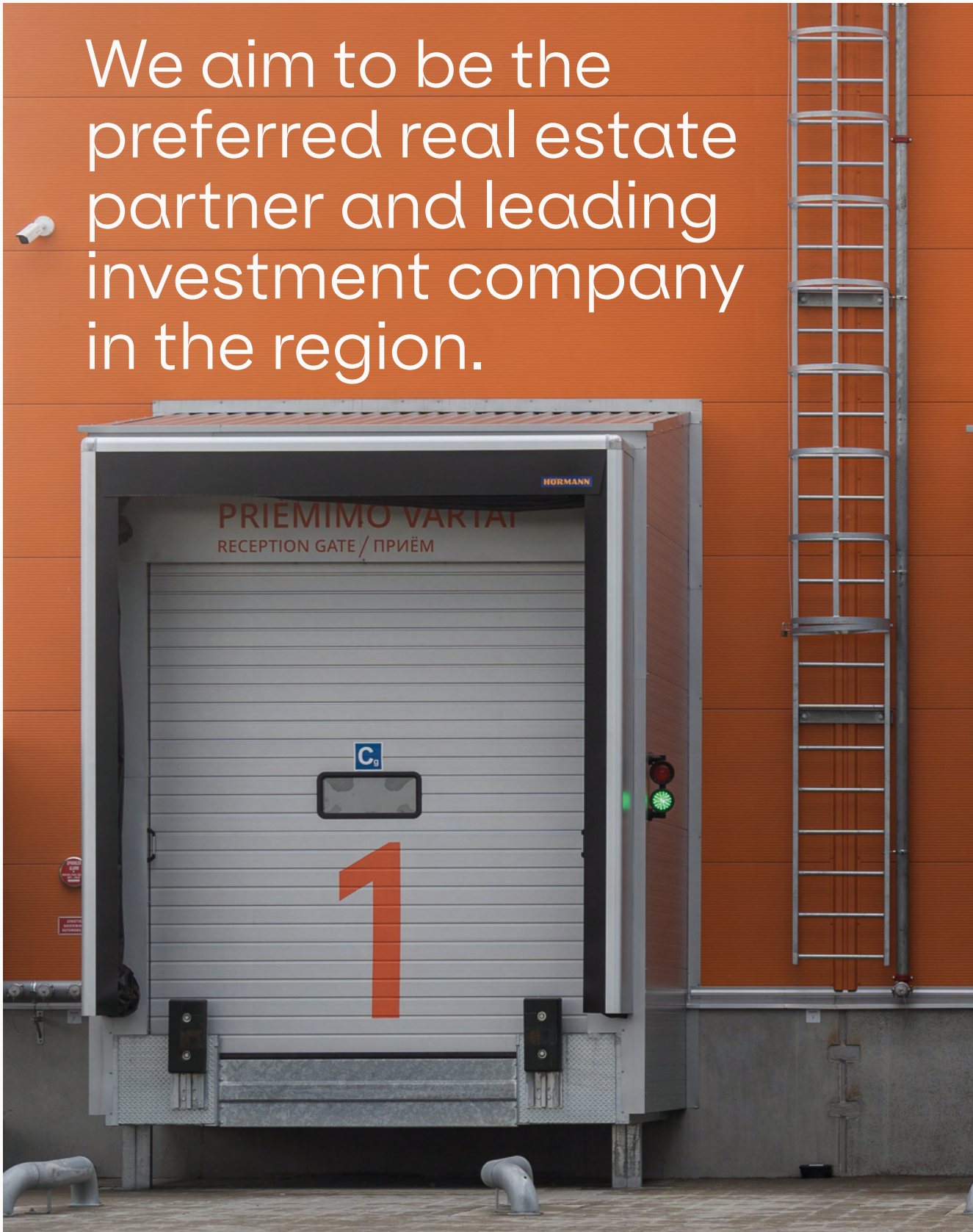
Oribalt terminal | Highway A1, near Vilnius
