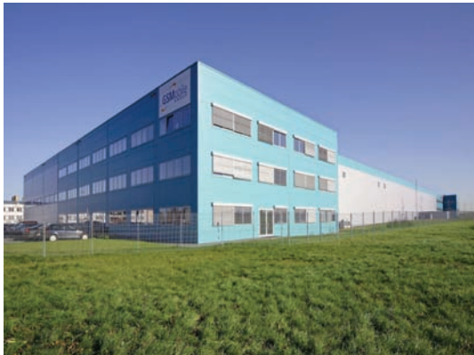
Project: Green Park, Prague - Letnany Tenant: GSMobile Group
