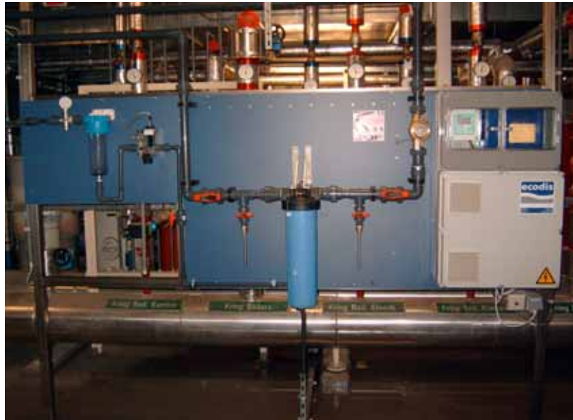
Typical installation: 1 cell of 4 m 3 /h placed in bypass of the main pipe for treating a total water flow of 20 m 3 /h.
