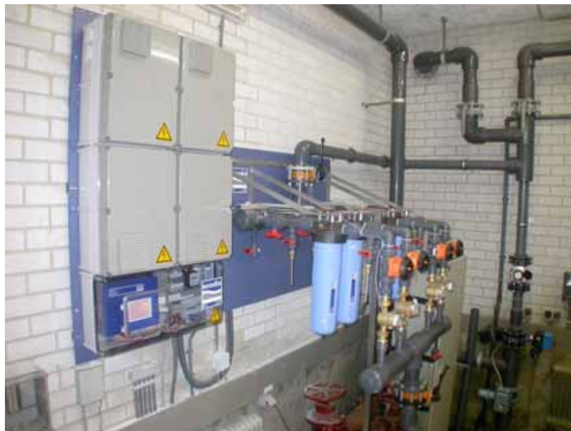
Typical installation: 4 cell of 5 m 3 /h placed in bypass of the main pipe for treating a total water flow of 40 m 3 /h.
