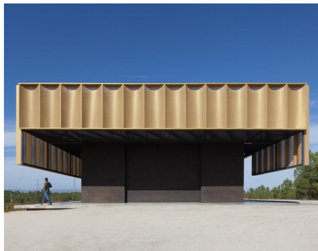
Adegas 23 lined with expanded cork agglomerate. A project by Rua Studio
